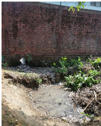
o) Digging of waste water outside the women's hostel
