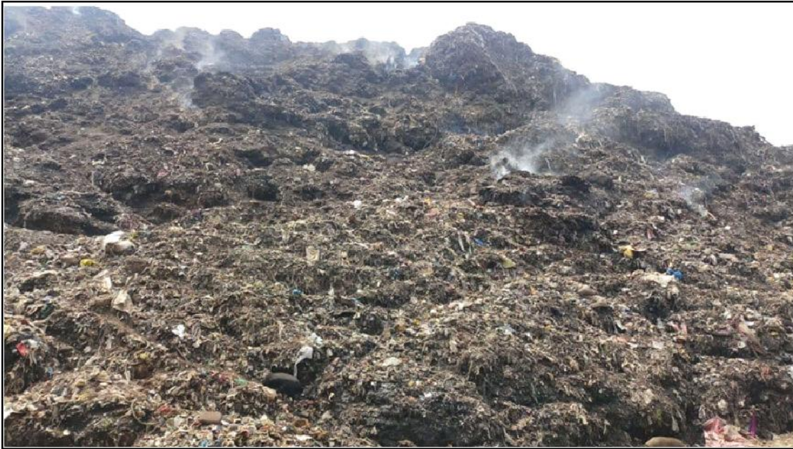
Fig.8 :The deplorable condition of the Dhapa Landfill (Source: https://citizenmatters.in/kolkata-solid-waste-management-dhapa-howrah-belgachhia-landfills-segregation-12951 )
